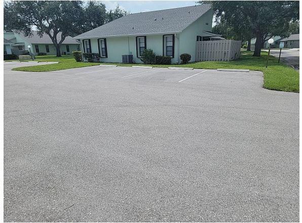
Asphalt street and parking
