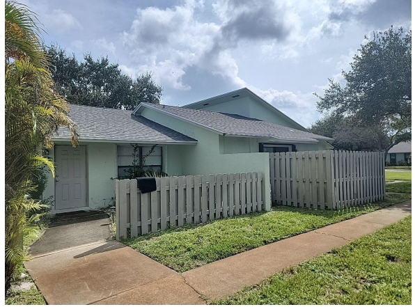
Example of Dwelling building - rear
