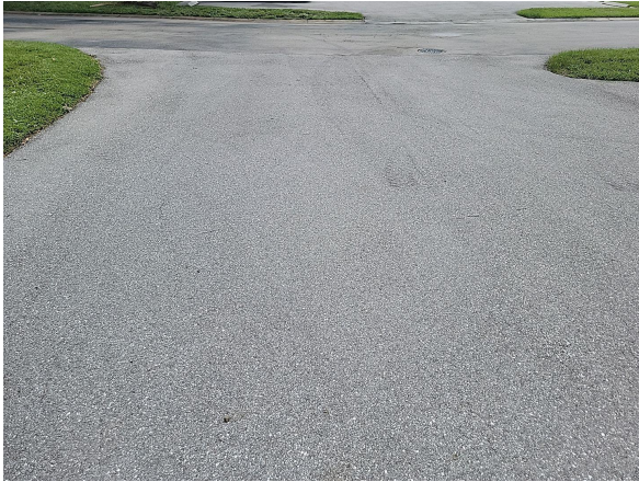
Asphalt paved parking
