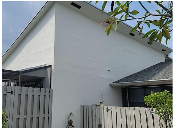
Wavy stucco siding
