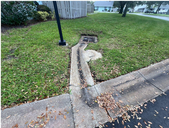
Damaged culvert
