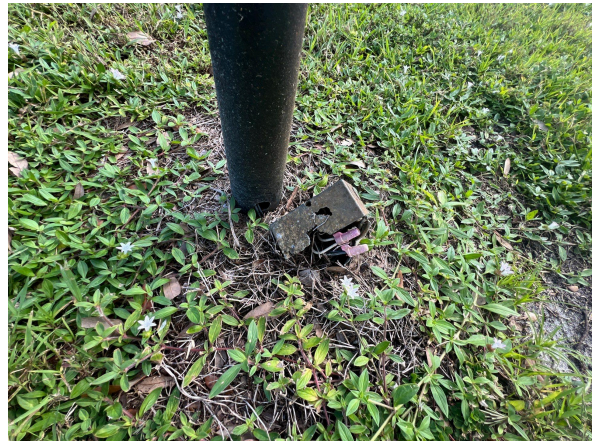
Exposed electrical wiring
