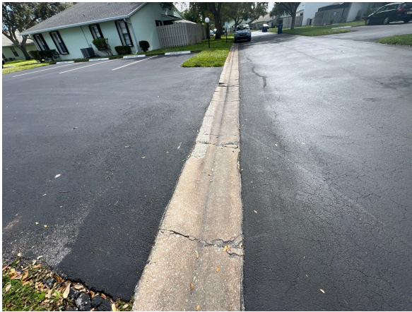
Damaged curbing/guttering
