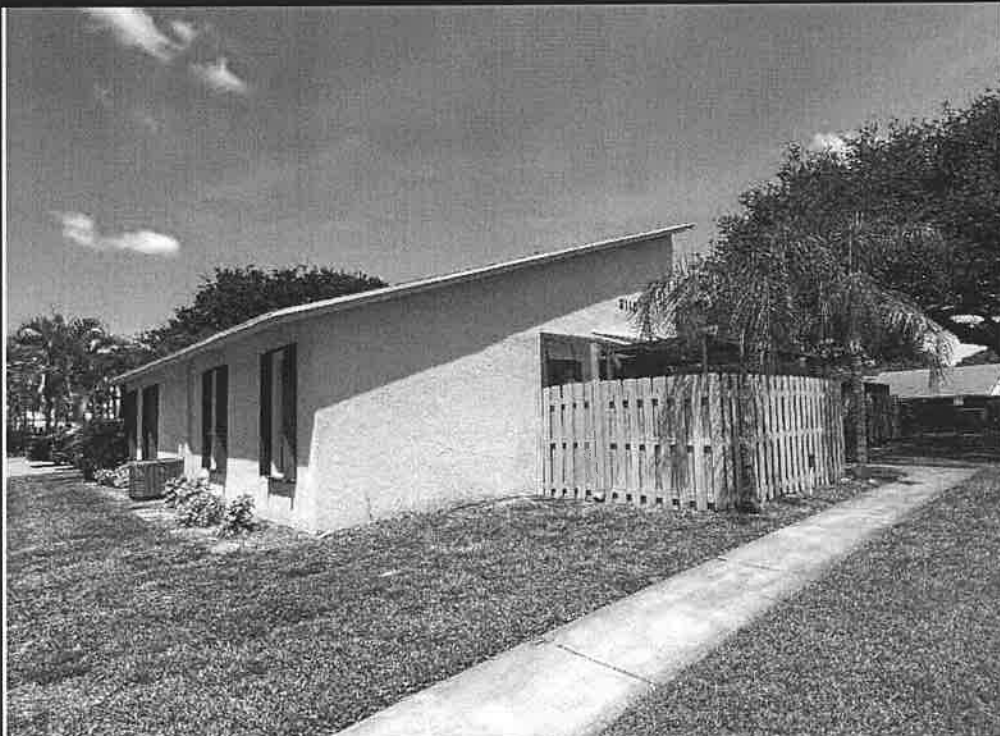
VIEW OF TYPICAL 4 UNIT BUILDINGS TYPE 1
