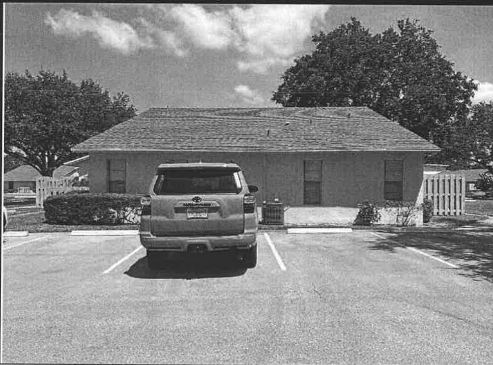
VIEW OF TYPICAL 4 UNIT BUILDINGS TYPE 11
