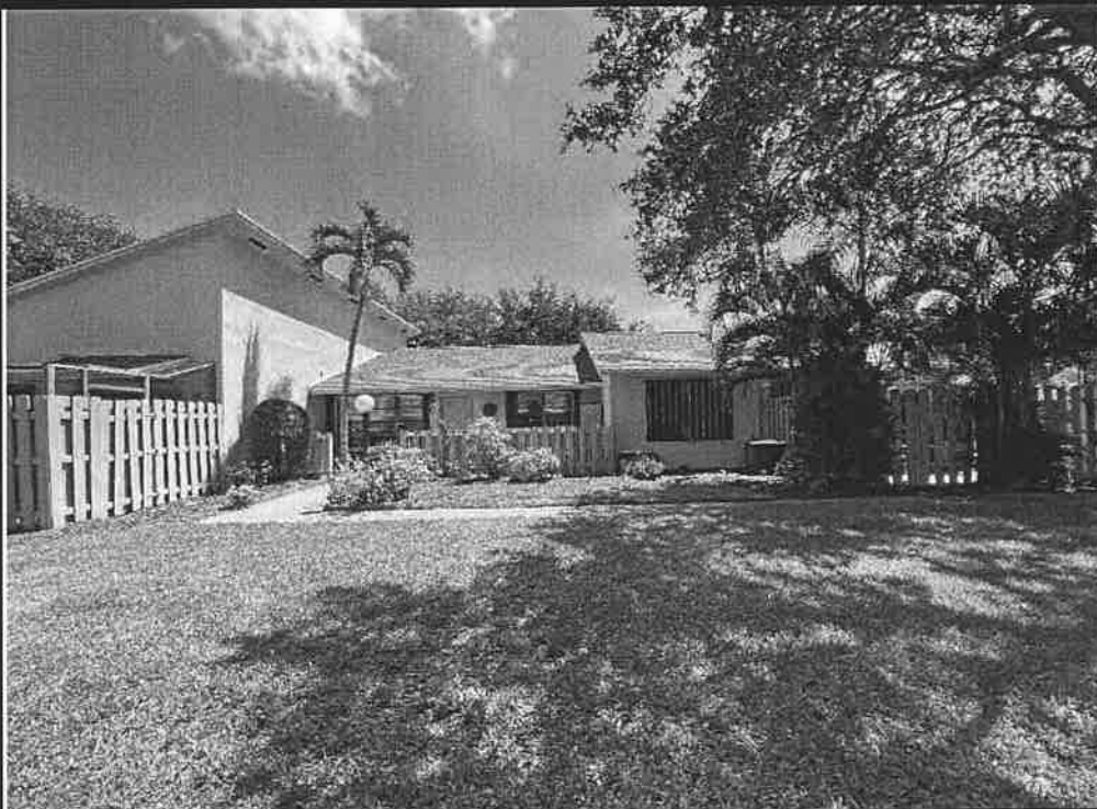
VIEW OF TYPICAL 4 UNIT BUILDINGS TYPE 1
