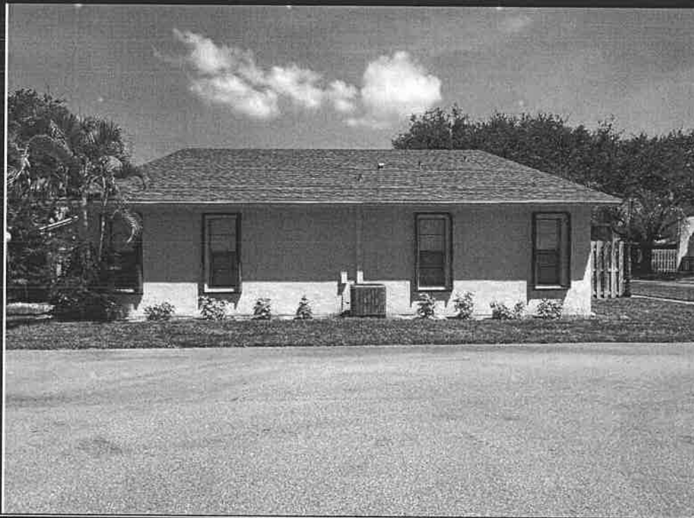
VIEW OF TYPICAL 4 UNIT BUILDINGS TYPE 1
