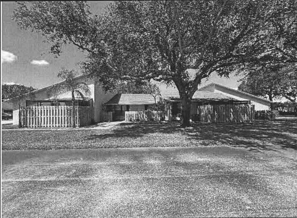
VIEW OF TYPICAL 4 UNIT BUILDINGS TYPE 1
