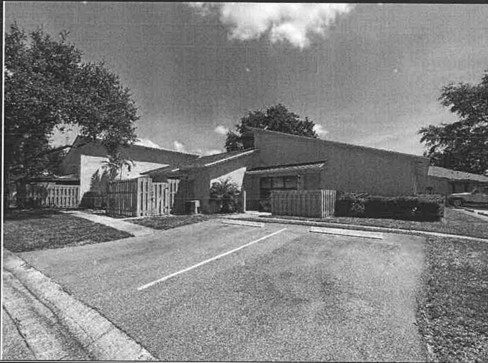
VIEW OF TYPICAL 4 UNIT BUILDINGS TYPE 11
