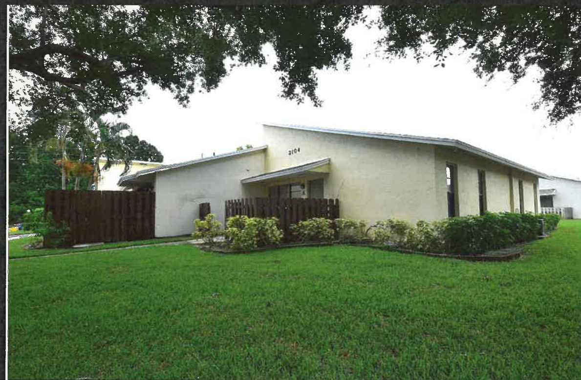
EXTERIOR VIEW OF TYPICXAL 4 UNIT RESIDENTIAL BUILDING
